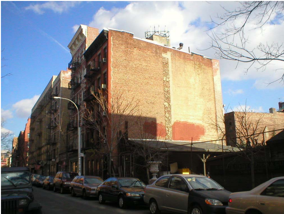
Figure 13. Adjacent Site Buildings - Mott Street (Author)
