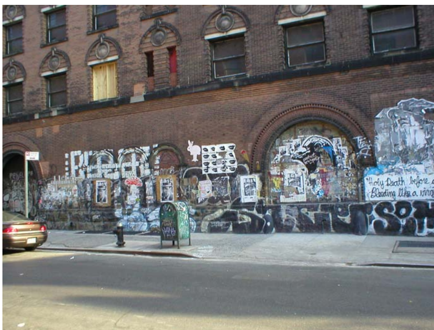
Figure 23. Building at corner of Elizabeth and Mullberry (Author)
